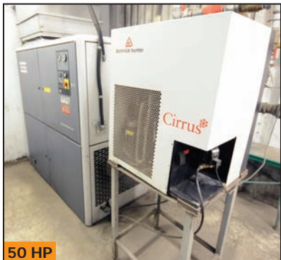
ATLAS COPCO rotary air compressor & air dryer
