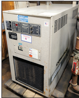
COMAIRCO SC250, refrigerated air dryer
