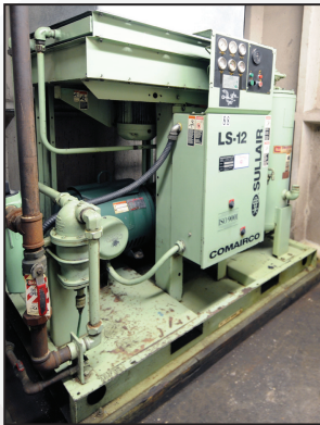
COMAIRCO LS12 rotary screw air compressor
