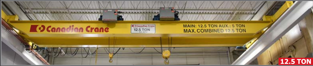
CANADIAN CRANE 12.5 ton double girder top running bridge crane
