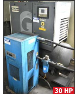
ATLAS COPCO GA22 rotary screw tank mounted compressor
