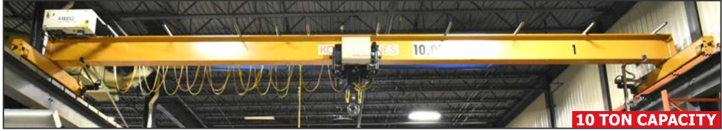
KONE single girder top running overhead bridge crane
