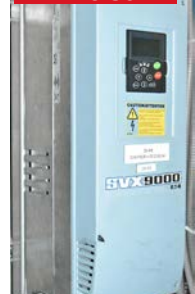
Partial view of EATON SVX VFDs
