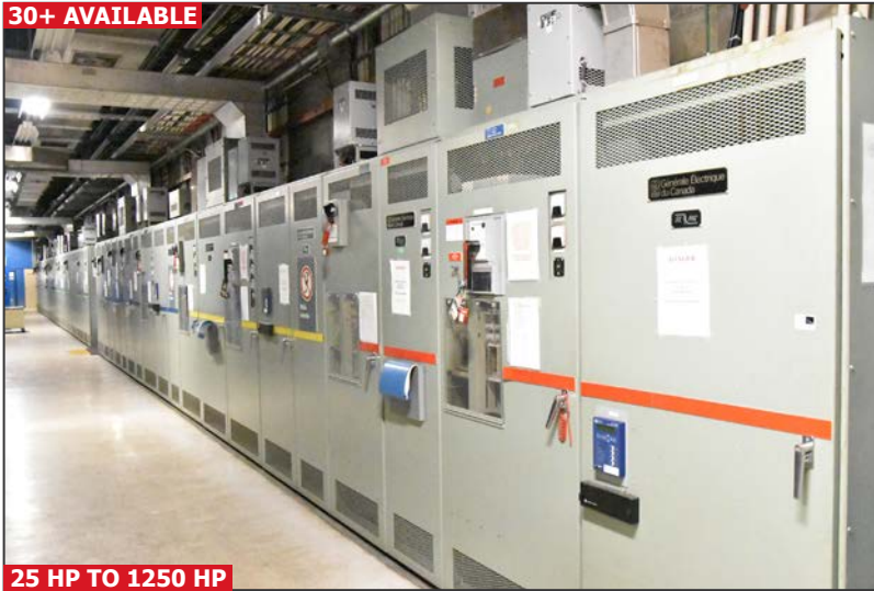
GE SILPAC VFD machine drive cabinets
