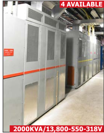
Partial view of POLYGON dry type transformers
