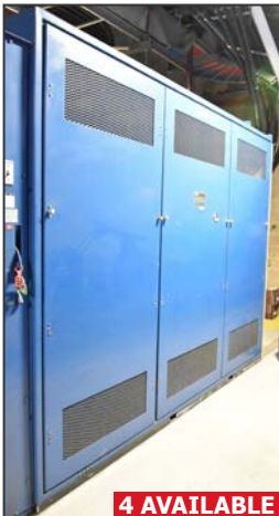
Partial view of BROWN BOVERI dry type transformers
